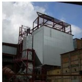
On Voskresensk cement plant successfully put into operation two electrostatic filter company FLSmidt Airtech (Denmark) for rotating kiln number 105 and 106.
